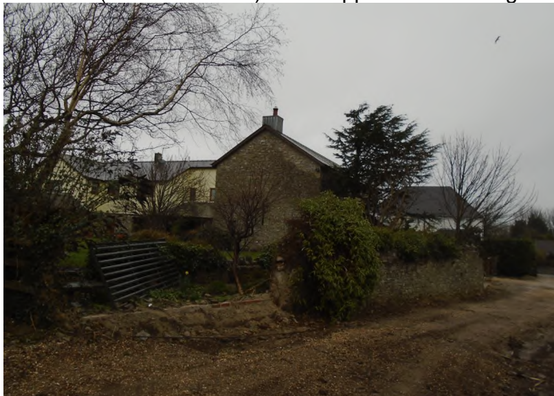
Rear (south elevation) of the application building
